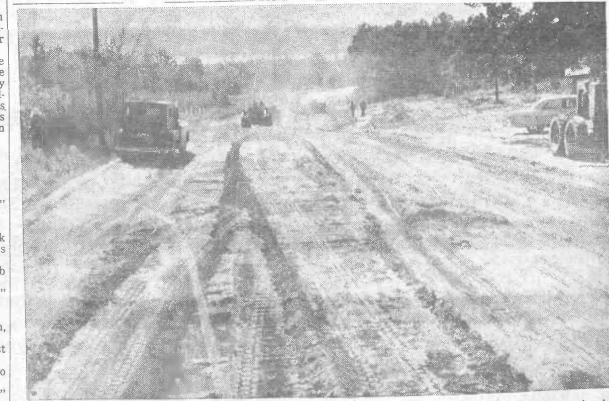
ROAD CONSTRUCTION—The above is a familiar scene in the northern part of the First Supervisor's District where a road to the new state park on Pickwick lake is now under construction. The above particular scene is the building of a cattle crossing under the new thoroughfare at the Albert Glover place. Mr. Glover is a grade-A dairy farmer and has lands lying on both sides of the road. The new road follows the old road generally. Widening of the roadway and straightening of the curves is some of the more noticeable improvements. New bridges are being installed, piling being driven in many places to give necessary strength. The road will lead from highway 25 east to the park.
